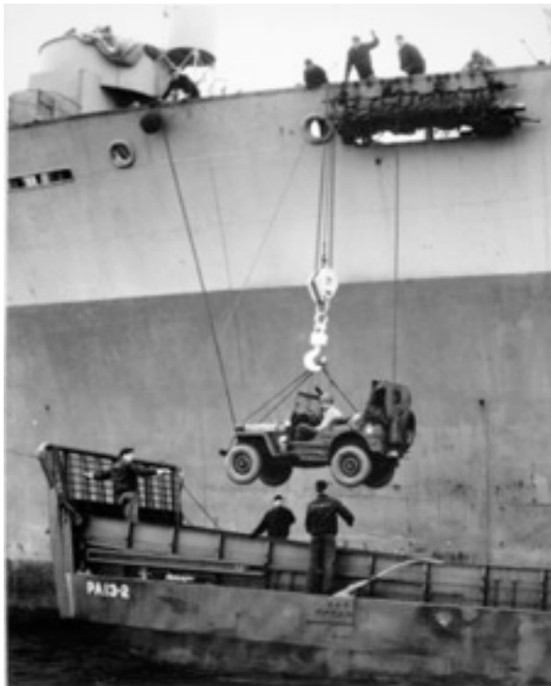
Figure 11. A U.S. Army Jeep is lowered into a landing craft in Normandy, 1944. The same methods were used in Guam. Photo from www.Olive-Drab.com , 2014.
