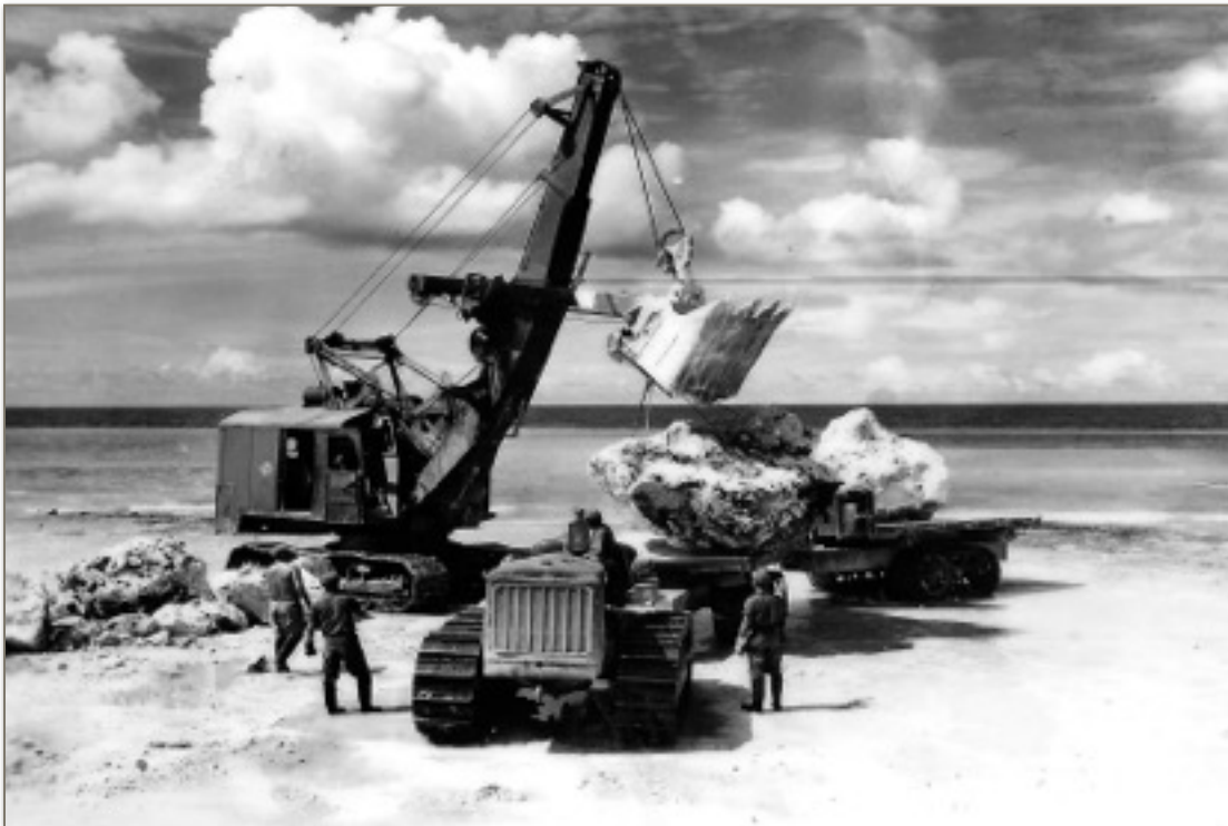
Figure 13. Building the breakwater. Courtesy James Oelke-Farley, National Park Service.
