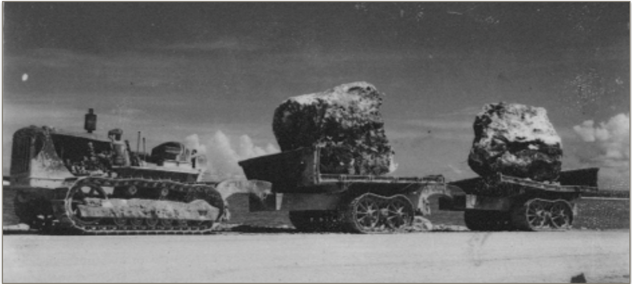
Figure 12. Building the breakwater. Courtesy James Oelke-Farley, National Park Service.
